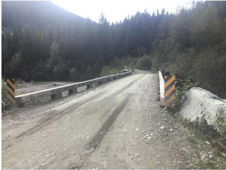
Approach from Left Bank when facing downstream
