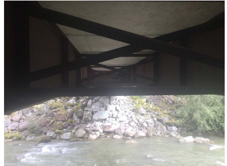
Left Bank Abutment when facing downstream
